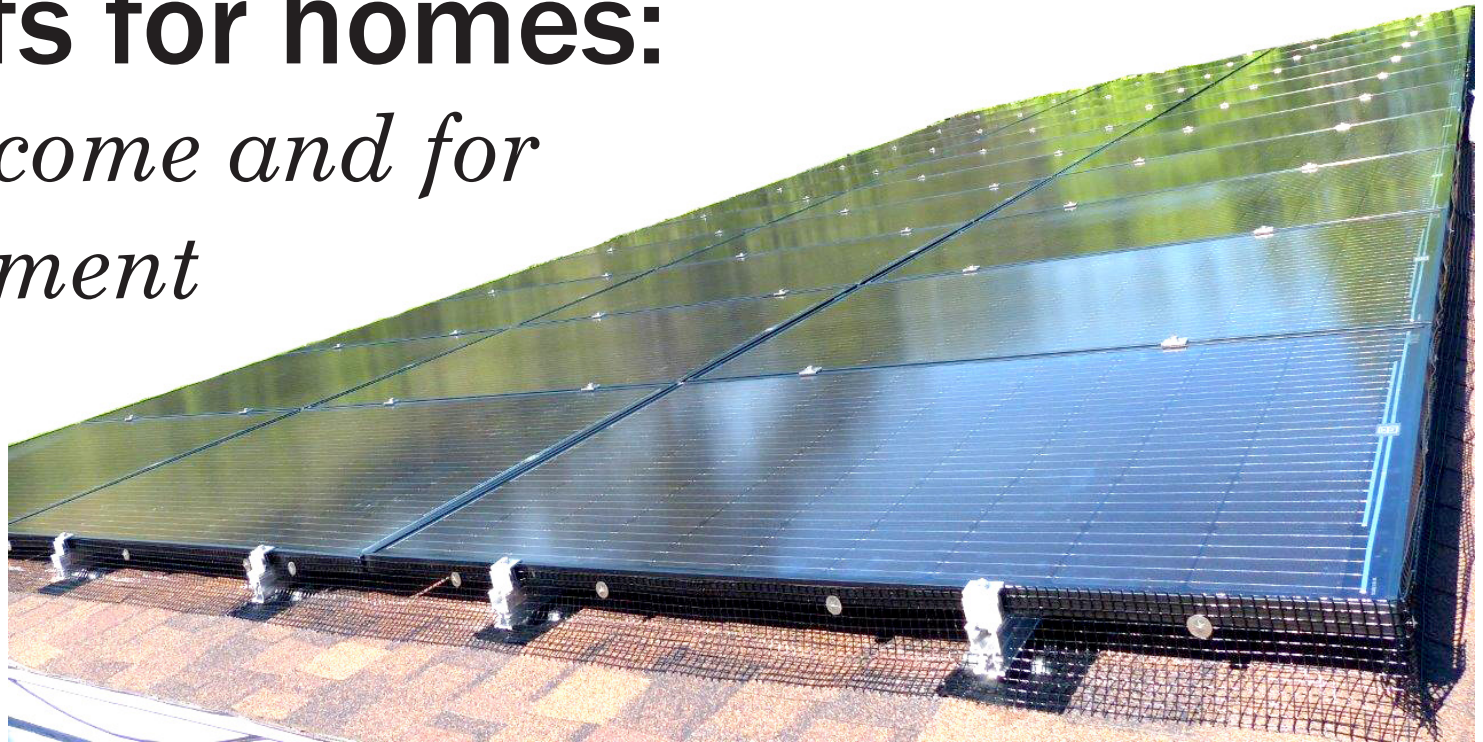
Josef Cihlar installed a 9.6 kW solar system on the roof of his home (pictured). The cost of solar technology has dropped dramatically in recent years giving small scale solar producers a 10% average return on their investment. Photo-Josef Cihlar.
